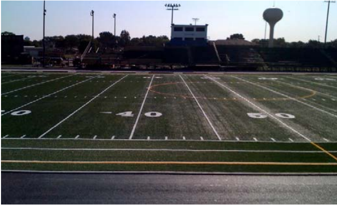
Final touches still required, but almost complete.
